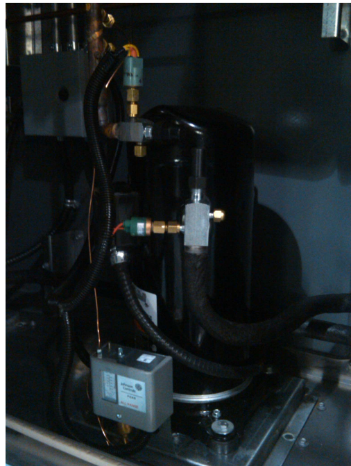
Digital Scroll Compressor
