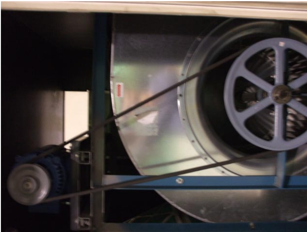
Figure 18: Blower Section
