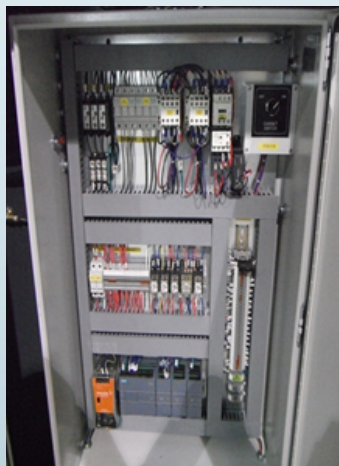
SEIMENS PLC WITH HMI
