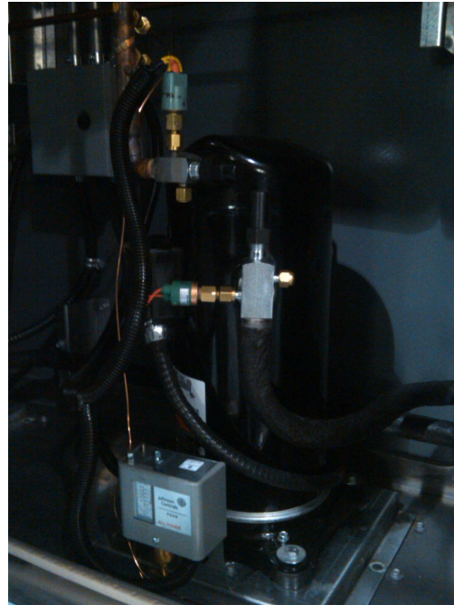
Digital Scroll Compressor
