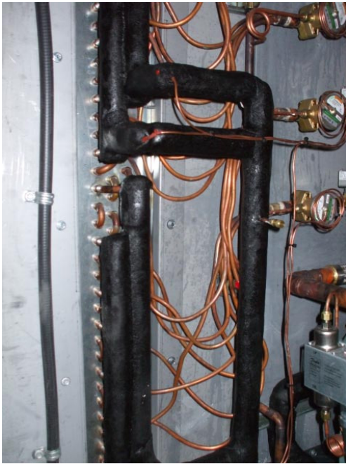
Figure 11: DX Coil Piping and Condenser
