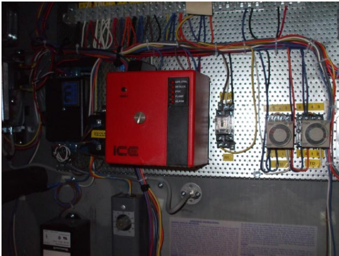
Unit Burner Proving System
