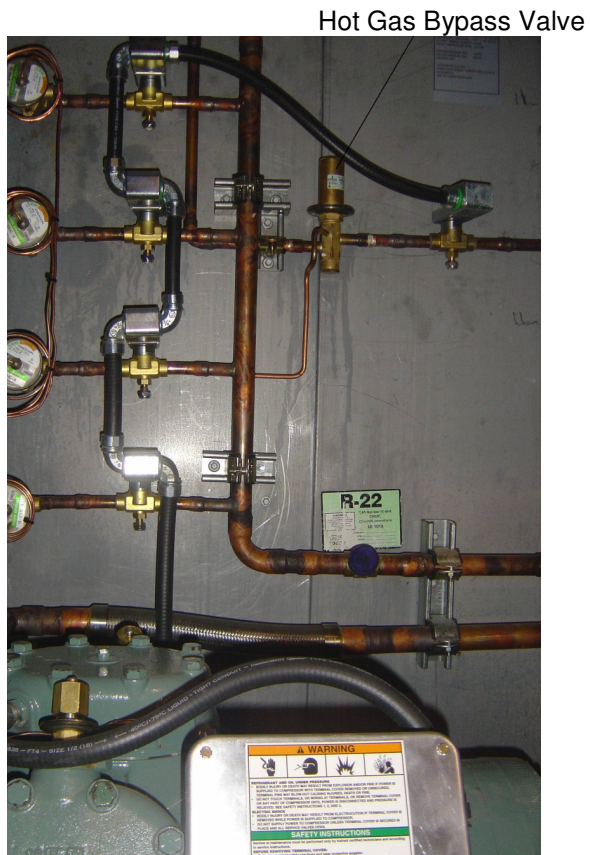
Figure5: Hot Gas Bypass System
